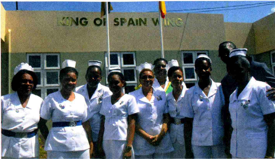
The refurbished wing at Spanish Town Hospital, a gift from the Spanish Government (Photo: Courtesy of the Jamaica Information Service)
